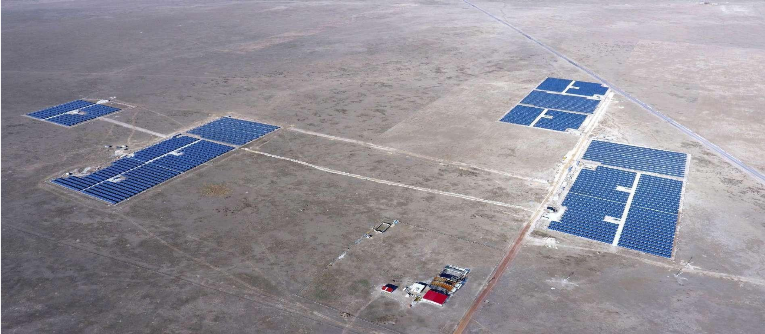
Niğde Bor Solar Park, 8 MWp, Turkey (2017)
